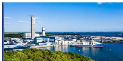
Figure 15: NKT's factory in Karlskrona, Sweden
