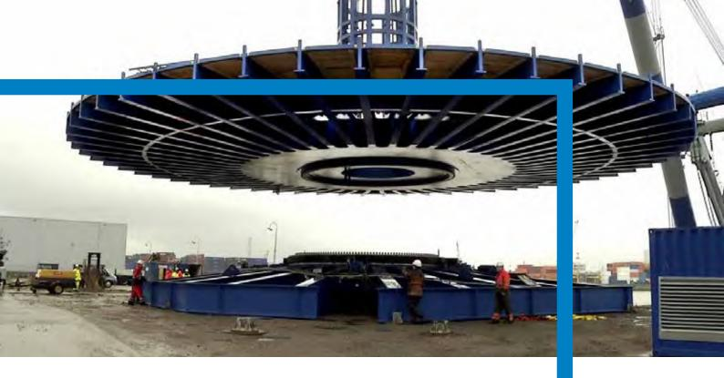
Installation of the turntable at the transhipment and storage terminal in Rotterdam which significantly increases the storage capacity for submarine cables.
